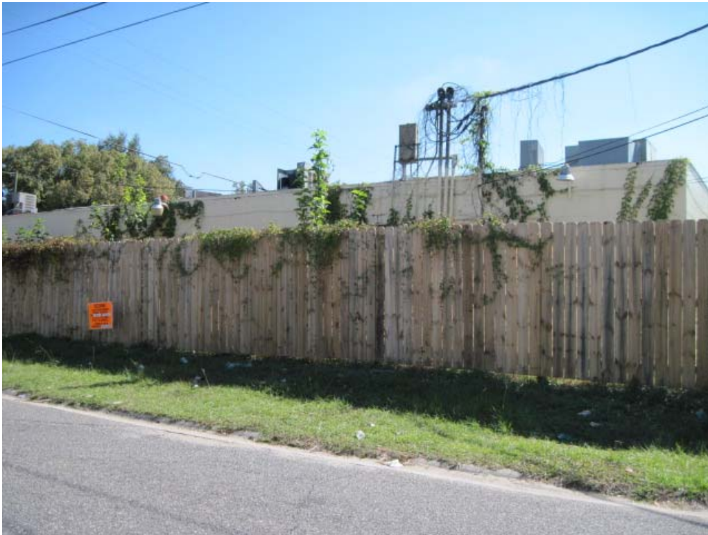
View of recently constructed wood fence along north property line.
