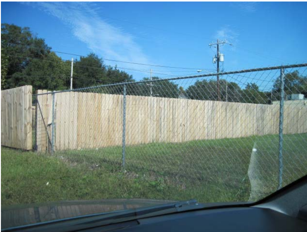
Recently constructed wood fence along west property line.
